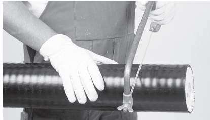
2 Cut the casing pipe with saw.
