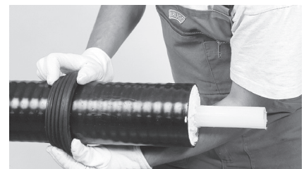
6 Install the wall sealing ring.
