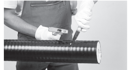
3 Split the casing pipe with knife. Note: Don't damage the carrier pipe!
